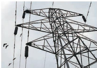
The pylons would be built in the Stour Valley
